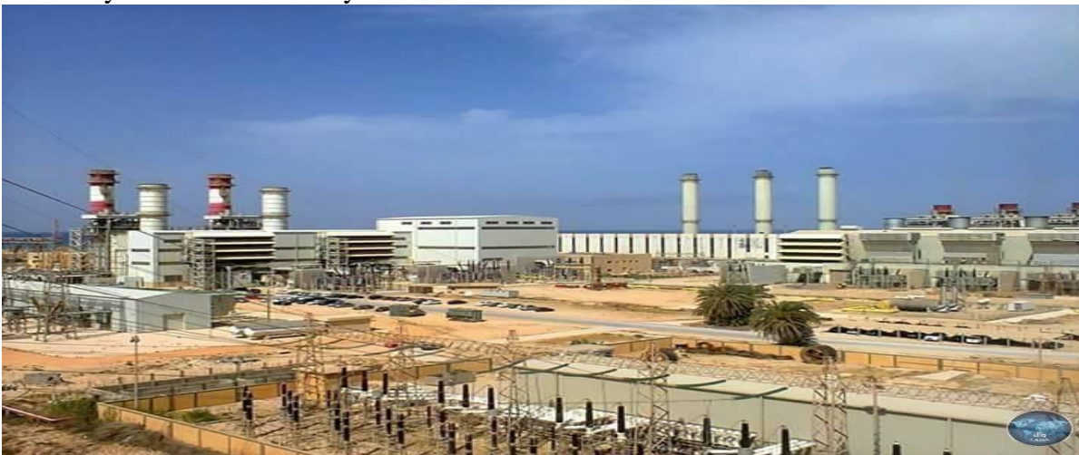
Figure 3. Benghazi combined cycle power plant
