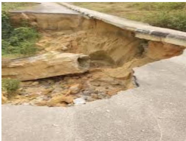
Fig. 3a. Road damage at Tombia caused by heavy Fig. 3b. ground damage near Tombia – Agudama vehicles laden with tonnes of sand Ekpetiama bridge caused by heavy vehicles laden with tonnes of sand
