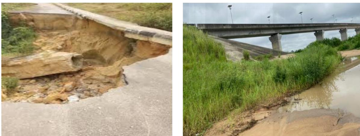
Fig. 3a. Road damage at Tombia caused by heavy Fig. 3b. ground damage near Tombia – Agudama vehicles laden with tonnes of sand Ekpetiama bridge caused by heavy vehicles laden with tonnes of sand
