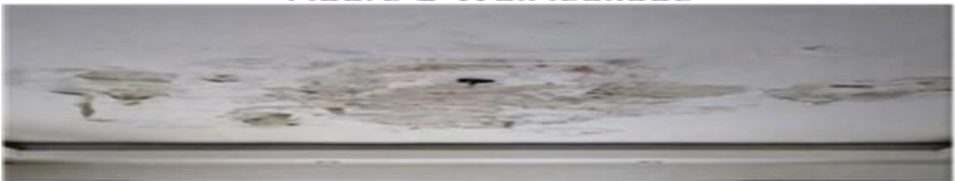
Figure 2: Roof leakage
