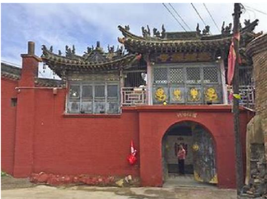
Figure 3: The situation around Datong ancient City Wall.
